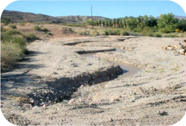
Pederson Channel construction © David Syzdek
