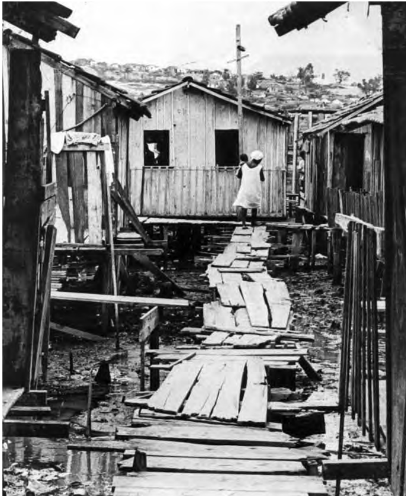
“Pontes de tábuas” (Wooden plank bridges) – Museu da Maré archives
