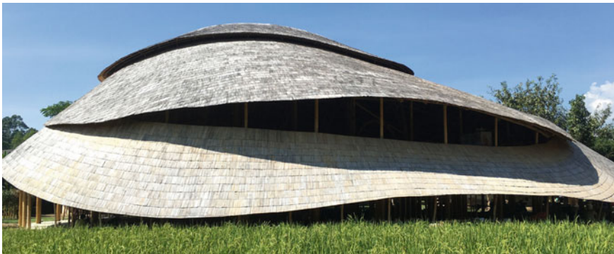
Fig. 10 Bamboo Sports Hall of Panyaden International School [35]
