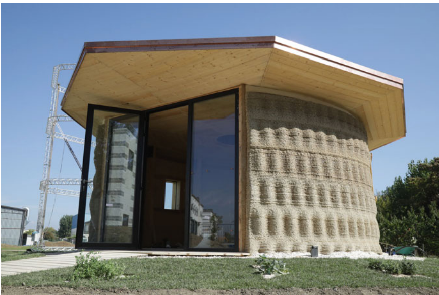
Fig. 8 3D printed the Gaia House [33]
