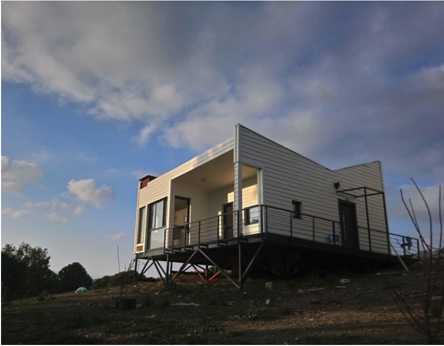
Fig. 3 A view of the low-cost ecological home
