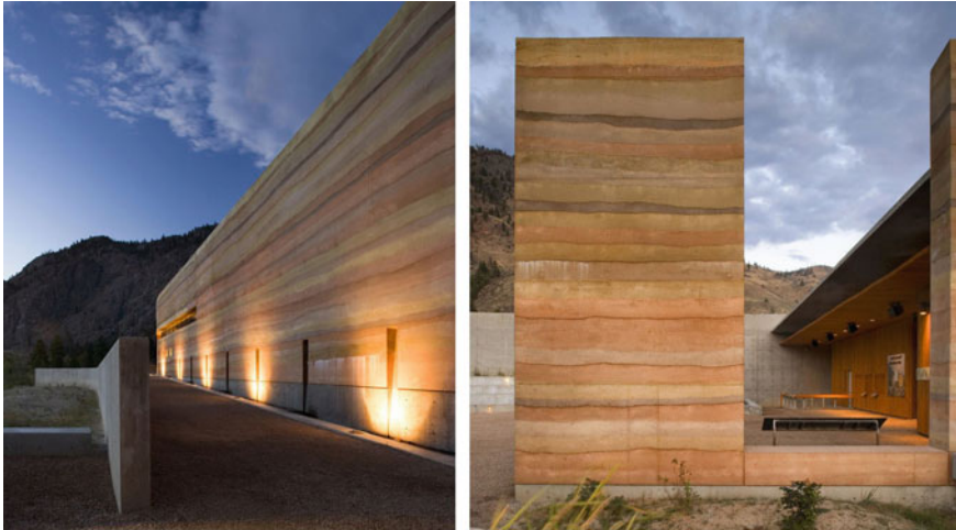
Fig. 12 Rammed Earth Walls of Nk'Mip Desert Cultural Centre [36]
