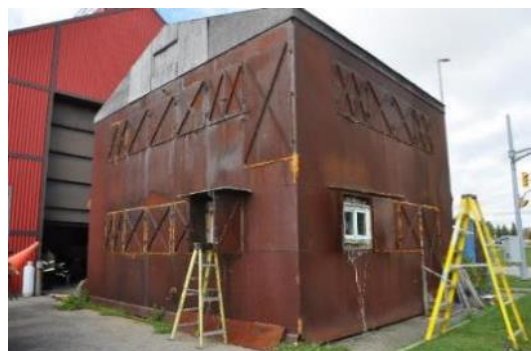
An external view of the burn house.
