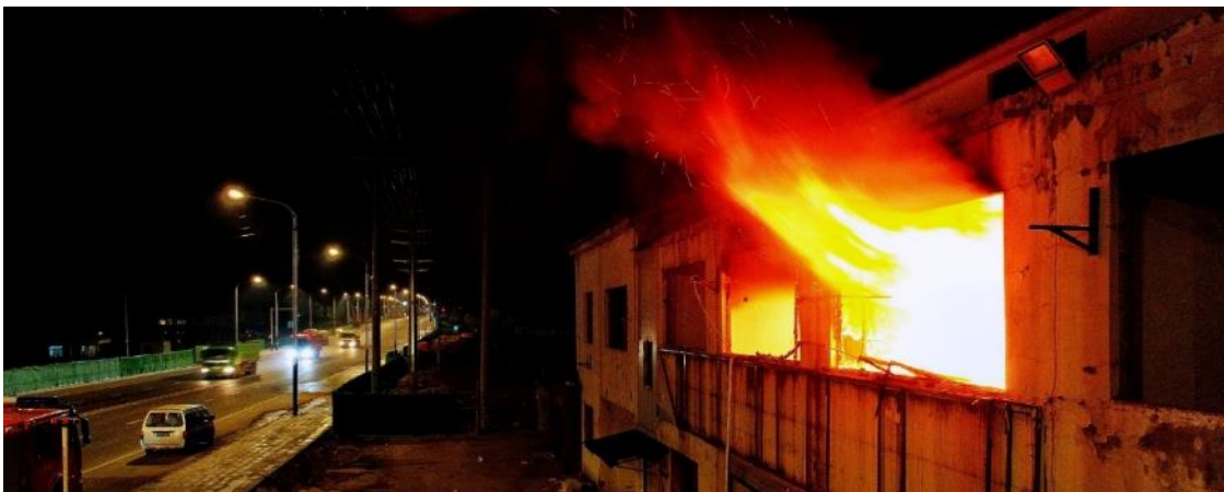
Ejected flame beside the road after complete fallout of window glass
